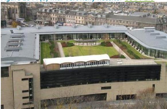
Figure 106 : (5) Toiture semi-intensive
