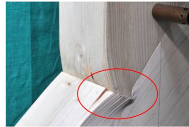
Crushing at the front-notch surface [1]
